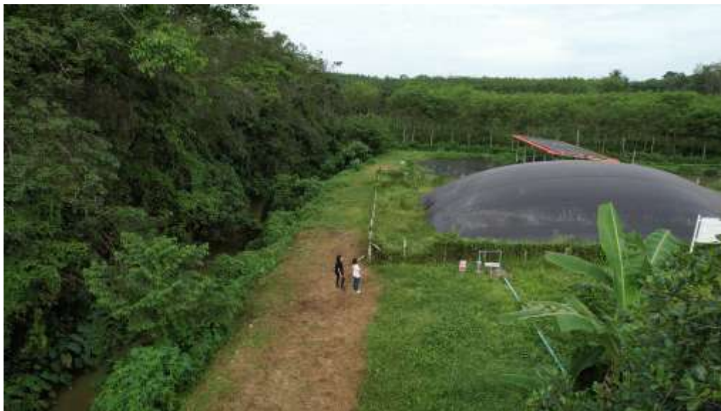
Figure 2. Installation of renewable energy and carbon offsetting scheme
